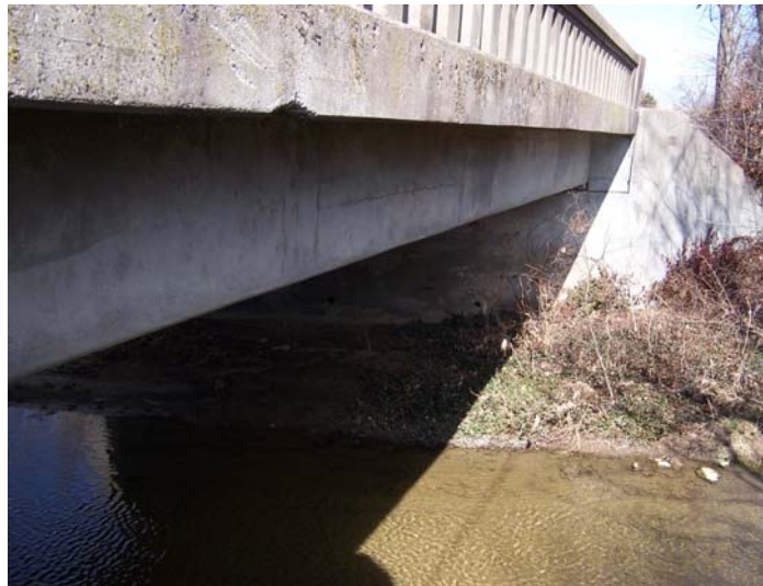
Figure 4: Bridge over Cartwright Creek (Pier and Beam)
