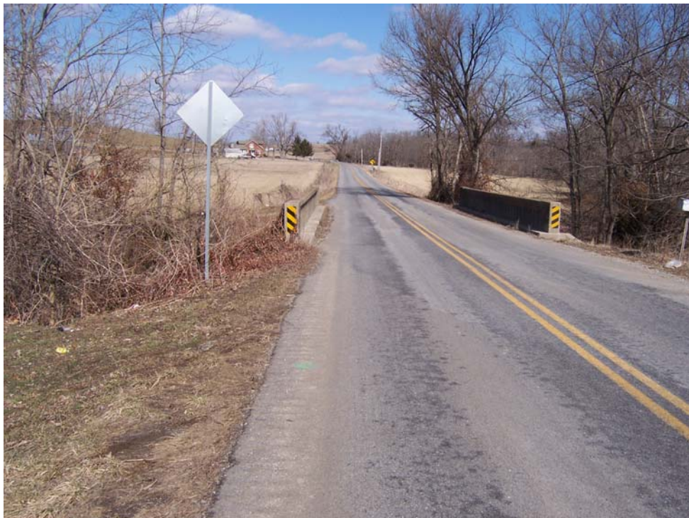
Figure 3: Bridge over Cartwright Creek Looking North
